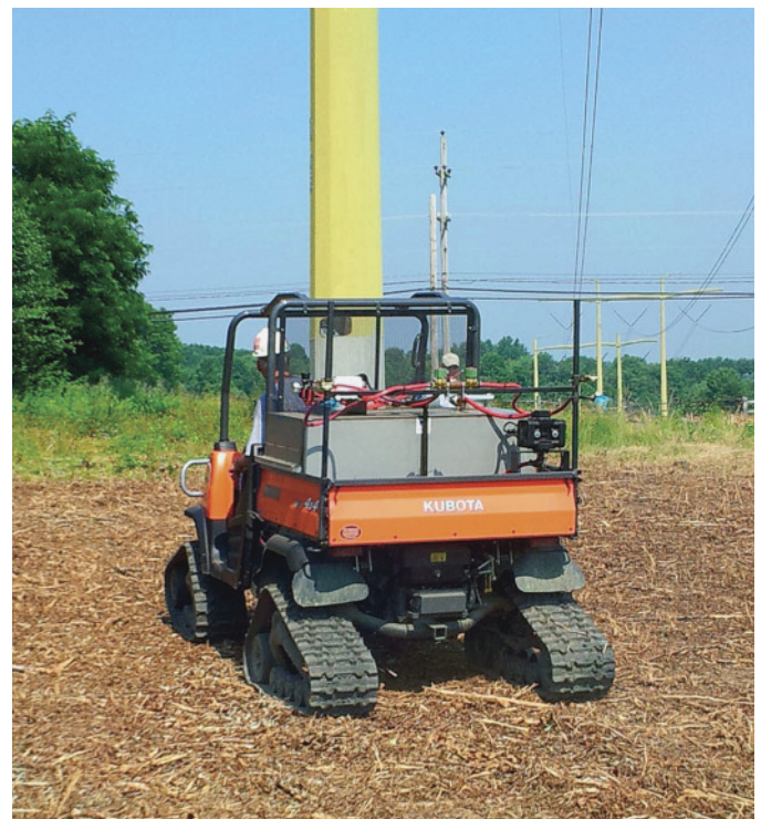
Photo 6 - Two THINVERT® Widecast™ nozzles mounted on a tracked Kubota can make quick work of a cut stubble application on a transmission ROW by spraying a 25 to 30 foot swath.
